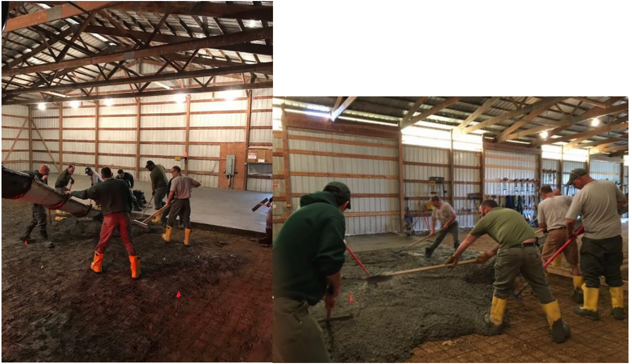
Trades and South Operations Staff pouring concrete floor. (Above).
