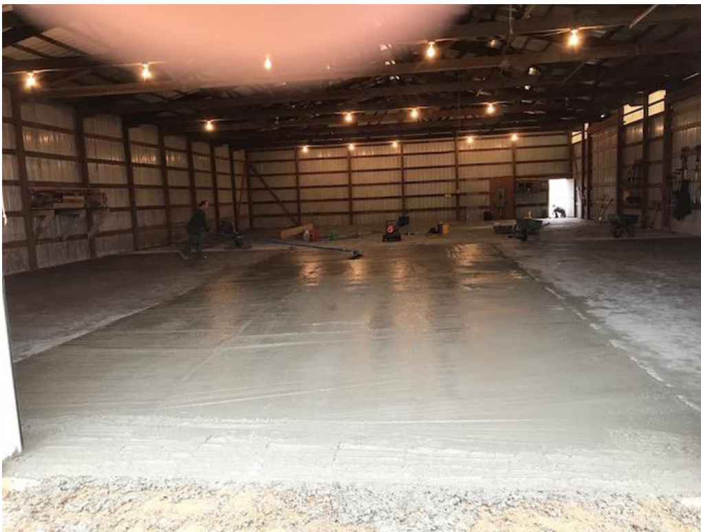
Completed concrete floor for the Grunwald Cold Storage Building.
