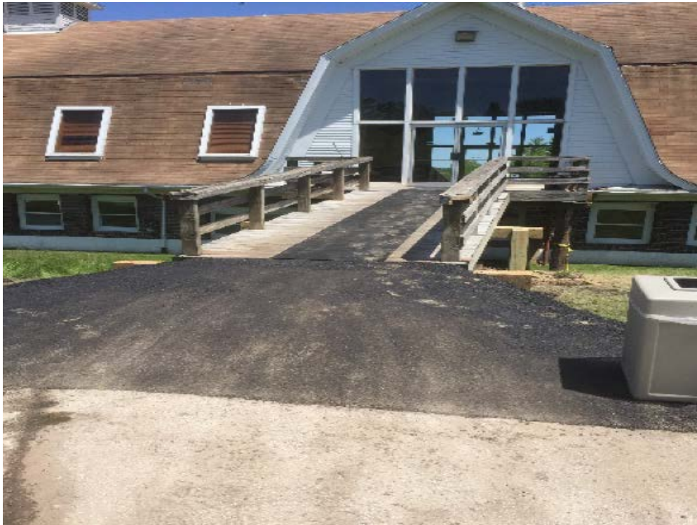
Settler's Hill Golf Course west-side entrance ramp repair.
