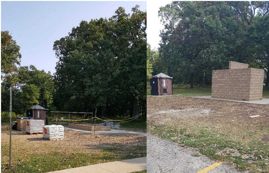
Photo of the start of the exterior restroom construction.
