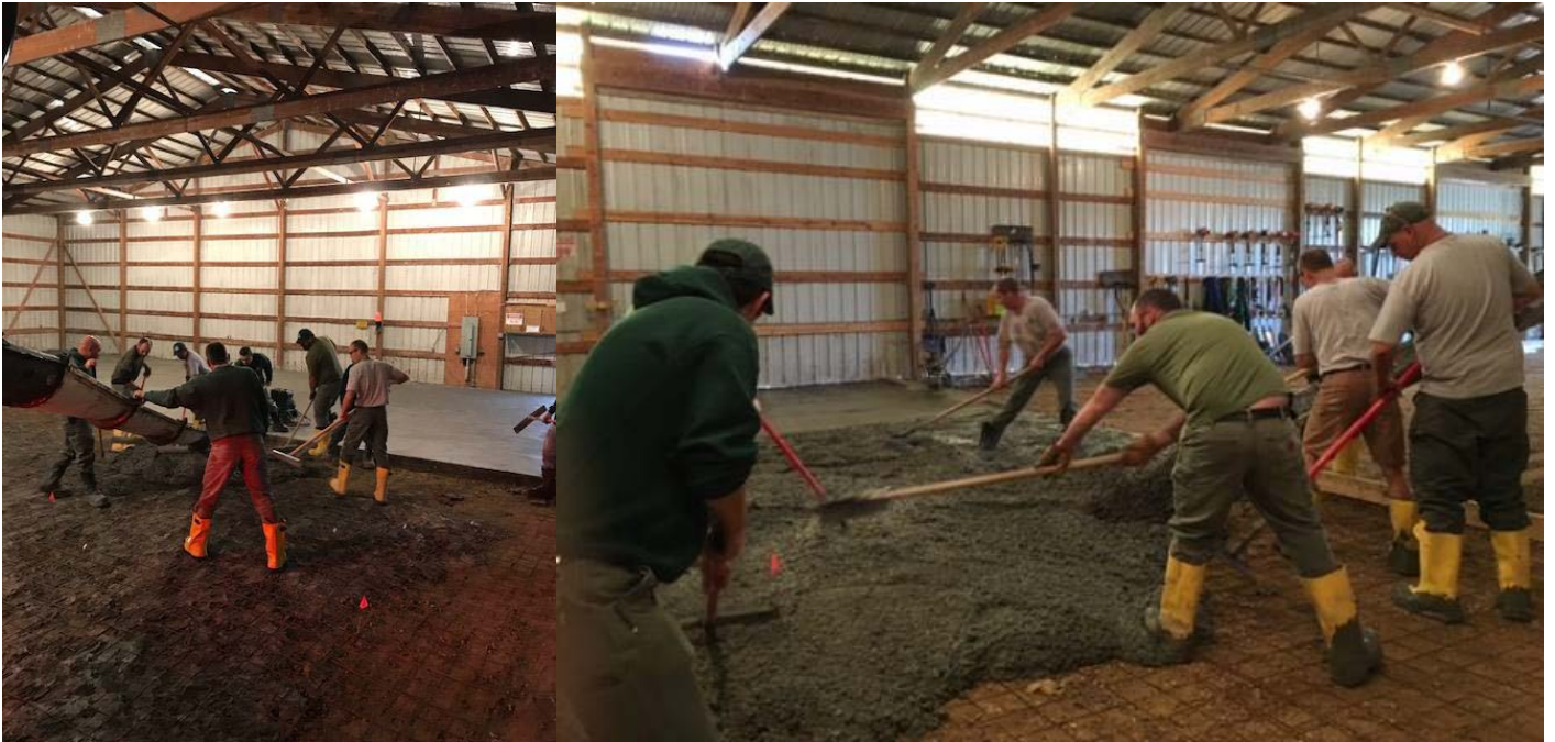
Trades and South Operations Staff pouring concrete floor.
