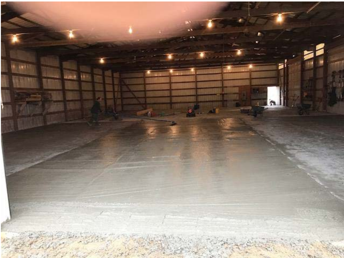
Completed concrete floor for the South Operations Cold Storage Building.
